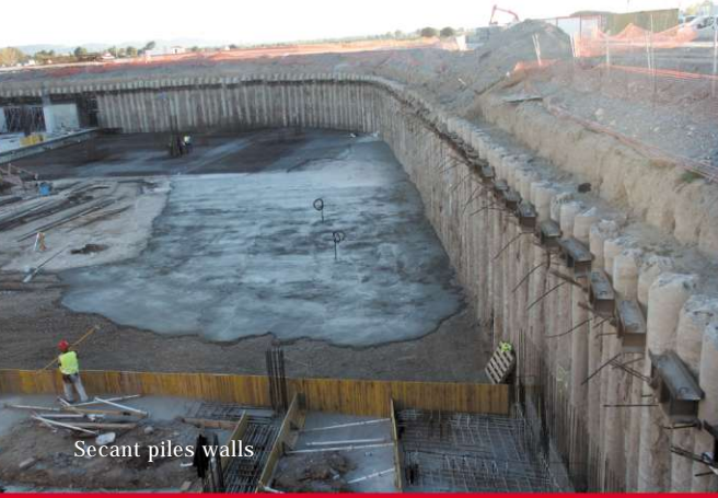
Discontinuous pile wall anchored in concrete capping and dividing beams
