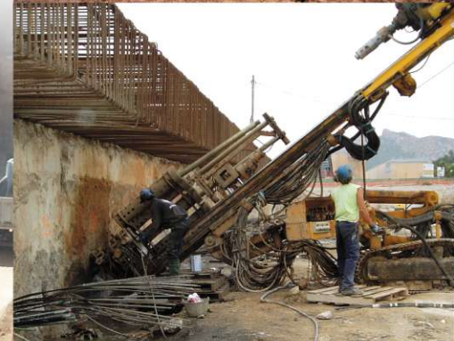
Multi-bulb anchors tested up to 200 t per anchor
