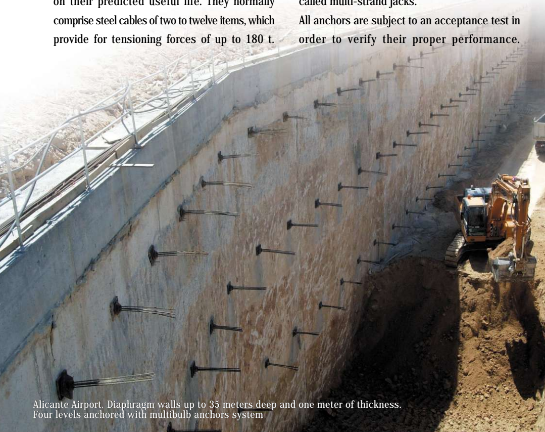
Multi-bulb anchors tested up to 200 t per anchor
