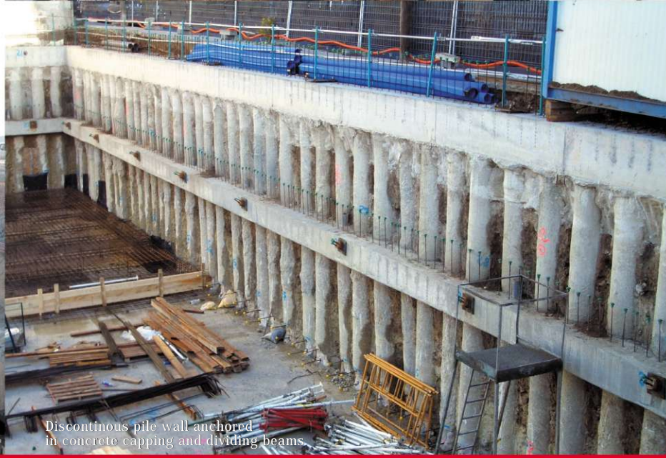
Anchored discontinuous pile wall for the new Mestalla Stadium, Valencia C.F.
