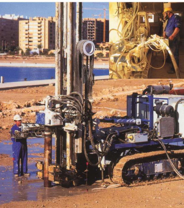
Alicante Airport. Diaphragm walls up to 35 meters deep and one meter of thickness. Four levels anchored with multibulb anchors system
